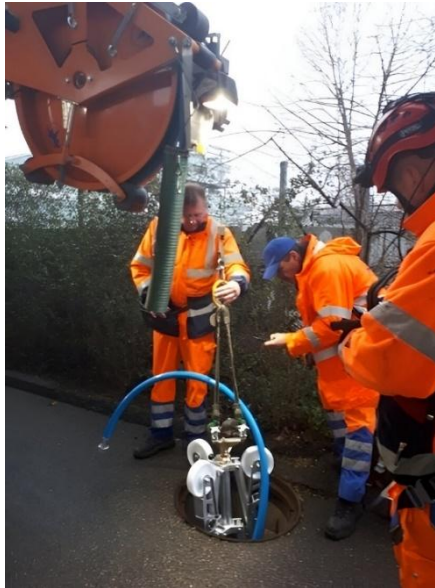
Figure 4 P360 being lowered into manhole
