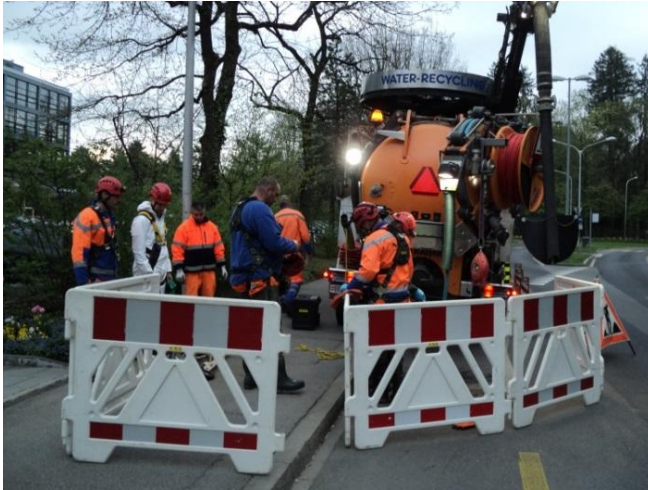
Figure 3 Cordoned-off & identified work area
