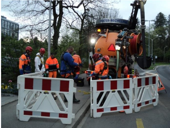
Figure 1 Blocked off & signed work area
