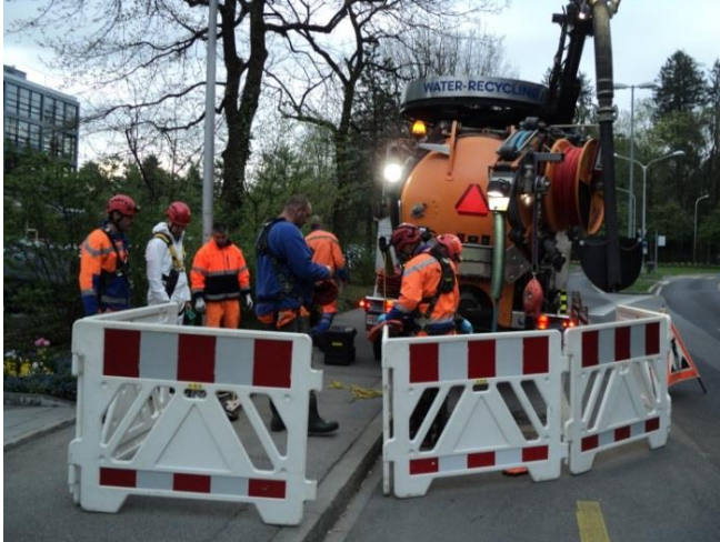
Figure 1 Blocked off & signed work area
