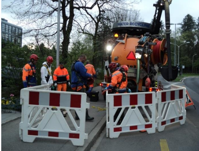
Figure 1 Cordoned-off & identified work area
