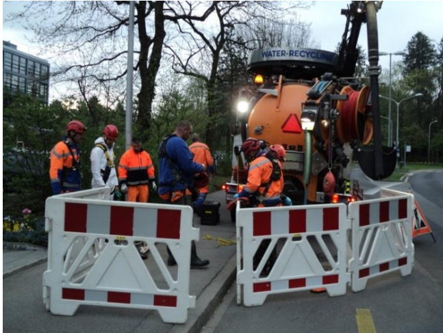
Figure 1 Blocked off & signed work area
