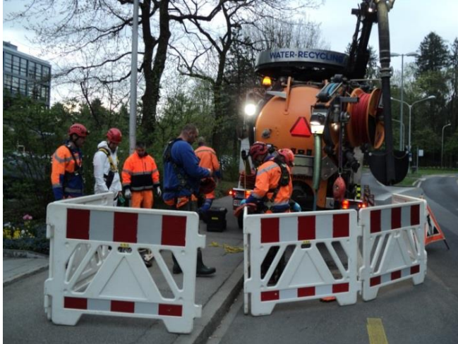
Figure 1 Blocked off & signed work area
