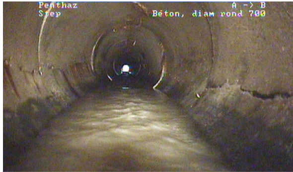
Figure 14 Damaged pipe wall
