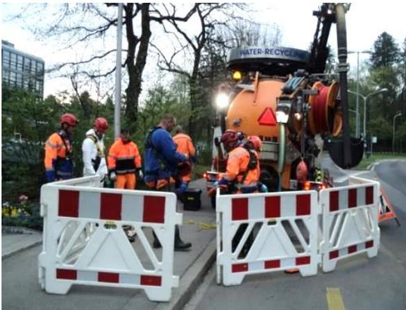
*Figure 10: Working area cordoned-off & marked*
